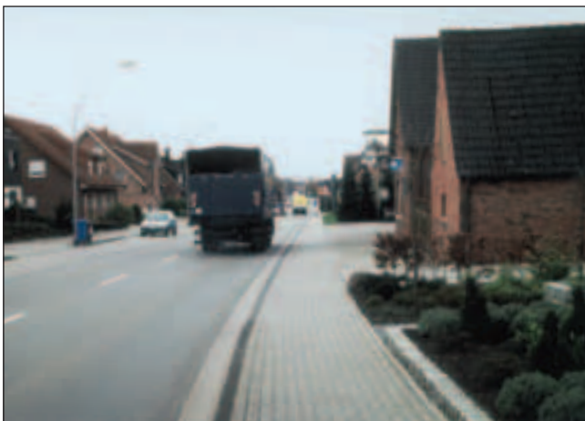
Condition of roads 2003.
