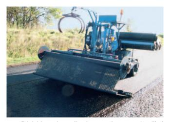
**HaTelit**<sup>®</sup> laid out immediately onto the sprayed, milled surface
